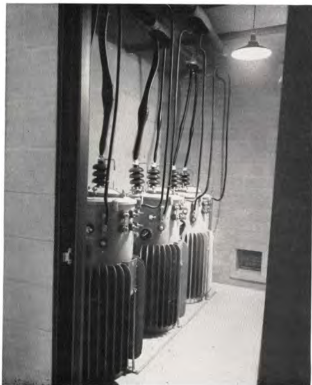
High voltage plate transformer vault.
