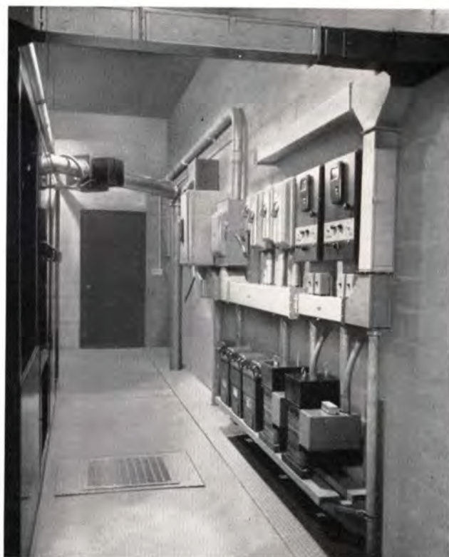
Typical arrangement of wall-mounted switch gear and distribution transformers. Door at rear gives access to the transformer vault.
