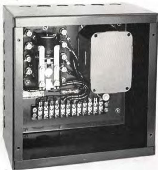
Tower Lighting Unit, MI-27519.
