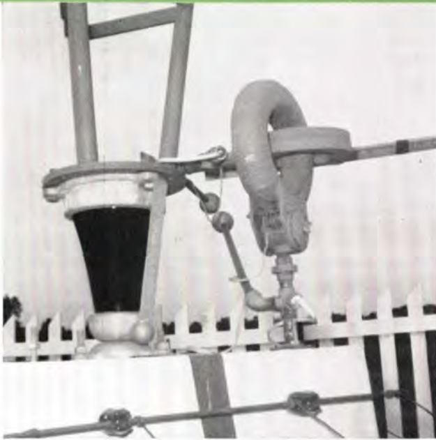
Typical installation of lighting transformer to isolate ac lighting circuit from rf.
