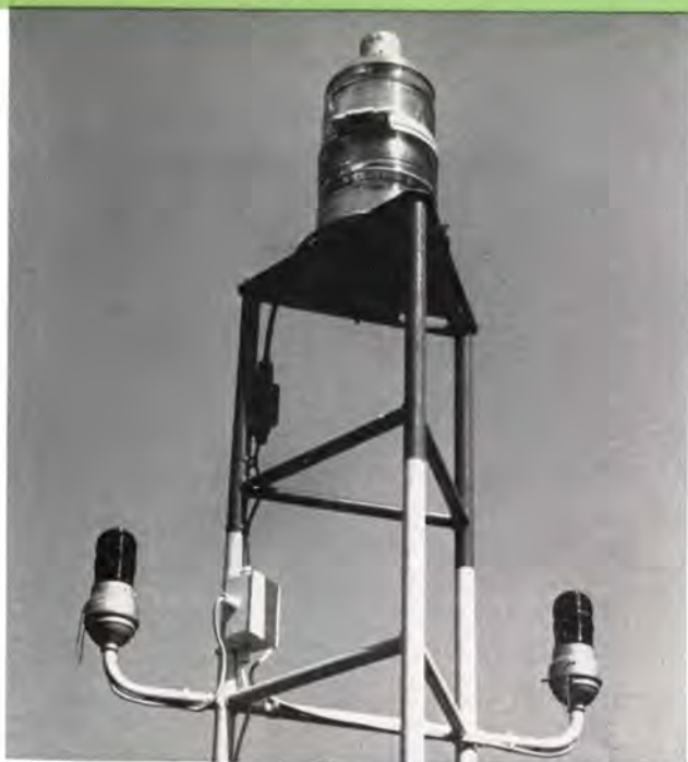
Main beacon and side obstruction lights shown powered by use of either lighting transformer or lighting choke coil.
