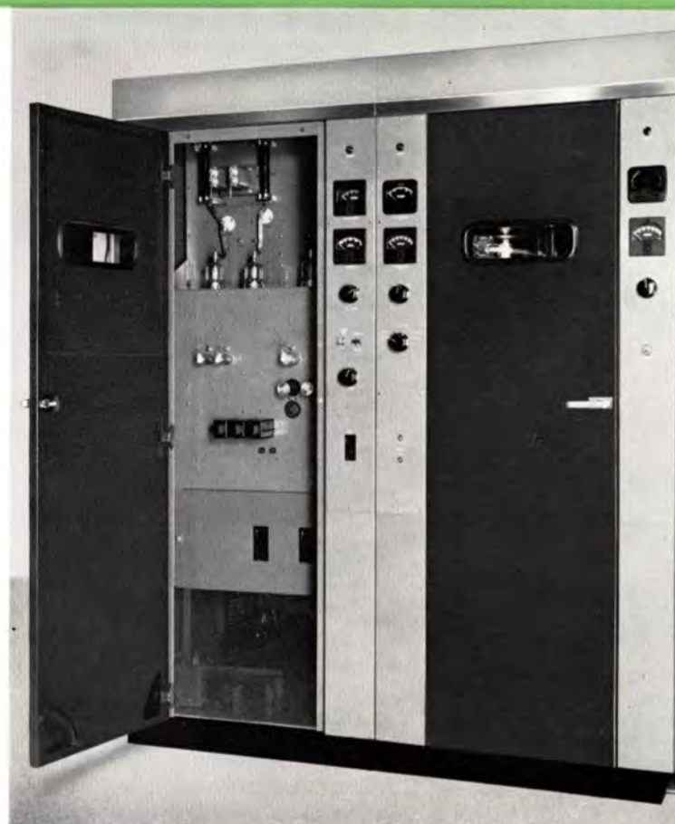
IPA and modulator driver stages of the BTA-5R can be seen at top of open cabinet. The exciter is at the center of the cabinet, and control equipment is placed just below the exciter.
